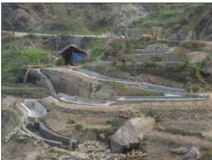
Figure 4. Linear type of raceway tanks for trout culture built by a farmer to fit the available landscape
