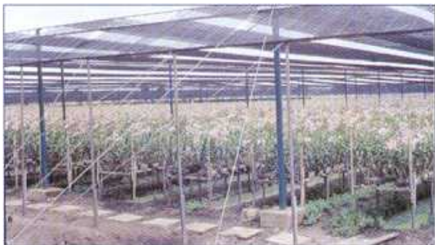
Greenhouse using galvanized pipes
