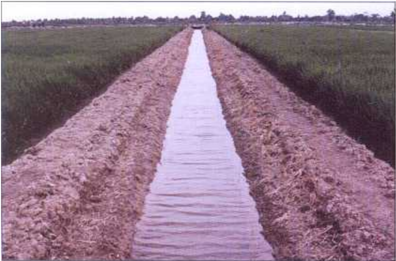
A vast area is covered under irrigated rice in West Java, Indonesia
