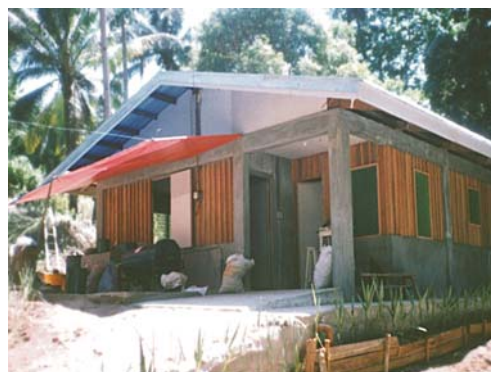
Figure 13. The newly established arrowroot processing plant.
